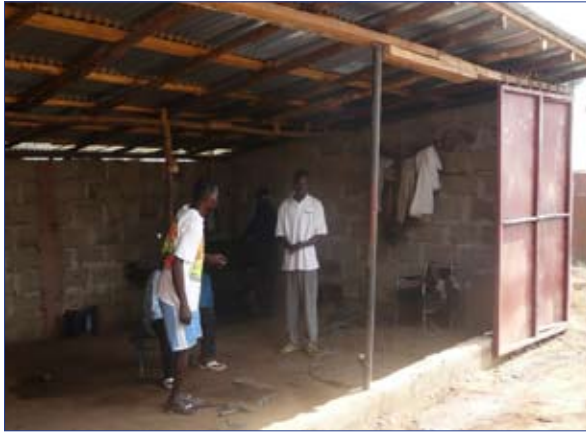
Left: The Welding Shed
